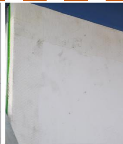
(c) Rasping of foam boards before application of base coat
