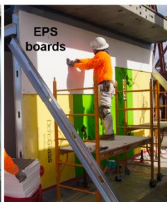
(b) Application of EPS foam boards using adhesive onto panel substrate
