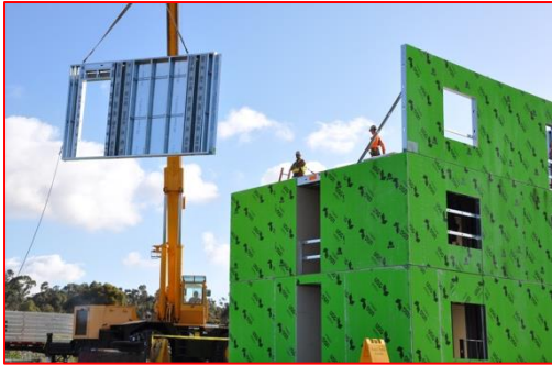
CFS-HUD pre-fabricated wall/floor panel (L2-L6) construction to LHPOST
