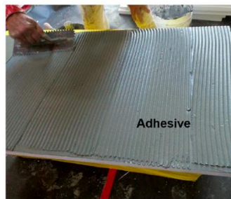
(b) Application of EPS foam boards using adhesive onto panel substrate
