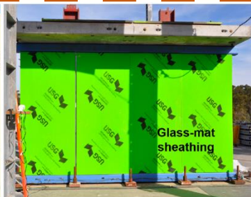
(a) Installation of glass-mat sheathing panels
