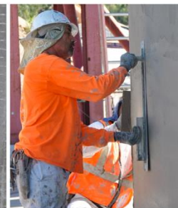
(d) Embedded reinforcing mesh in base coat and application of second layer
