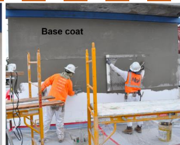
(c) Rasping of foam boards before application of base coat
