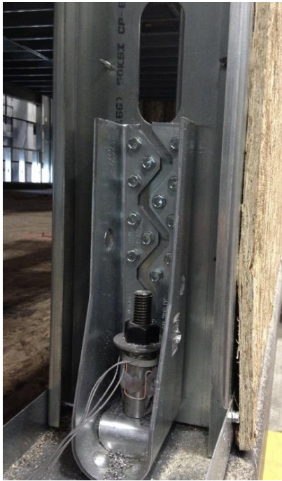
Hold-down on CFS chord stud ( CFS-NEES )
